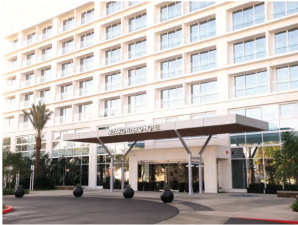
The energy-efficient Miyako Hybrid Hotel in Torrance, CA.
